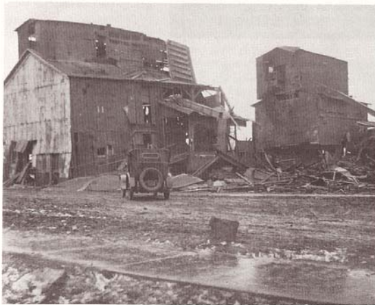
The old Auburn Rolling Mill after the explosion
